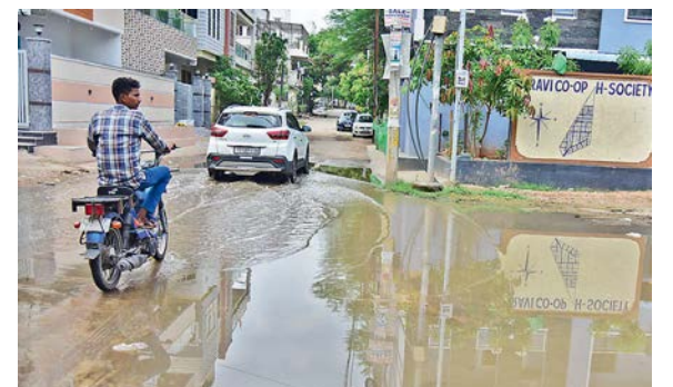
Rainwater stagnated on road at East Marredpally Ravi colony and Trimurti colony, which were dug up by GHMC authorities. —S. SURENDER REDDY
