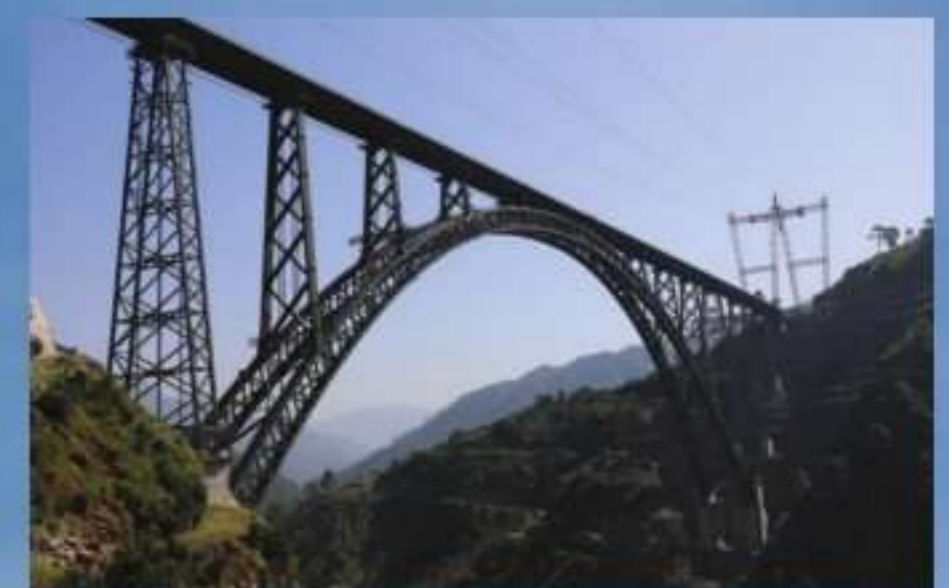
CHENAB RAILWAY BRIDGE, JAMMU & KASHMIR
