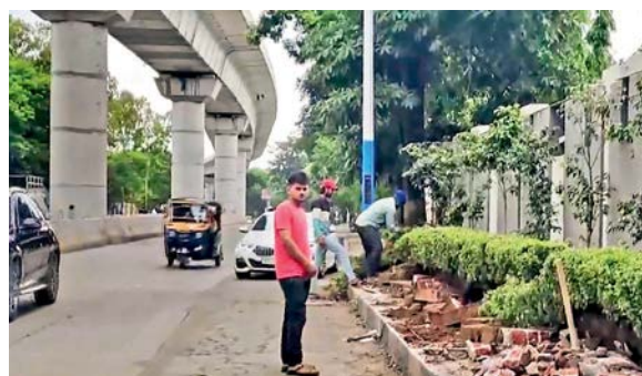
An illegal structure near trainee IAS officer Puja Khedkar's family bungalow being cleared, days after the Pune Municipal Corporation issued them a notice to remove it on Wednesday. — PTI
