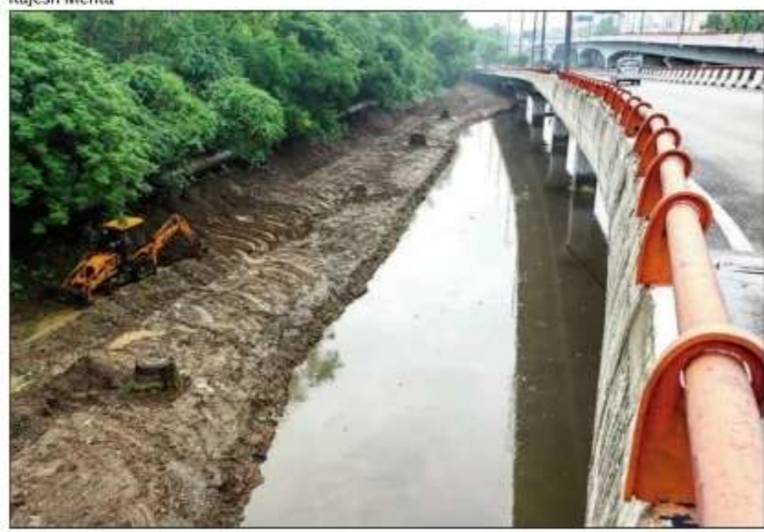
Preliminary desilting work is on at Barapullah and two key drains
