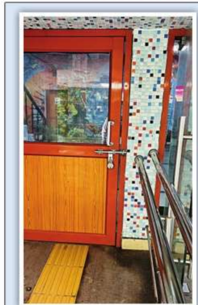
The building has a ramp, but the gate to its entrance remains locked
