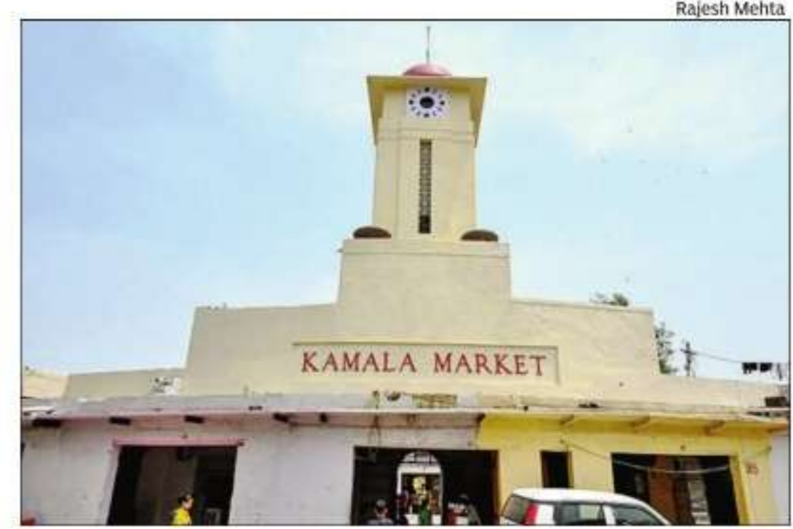
MCD had stopped the work after the repair and repainting of the clock tower due to the Lok Sabha elections and other reasons
