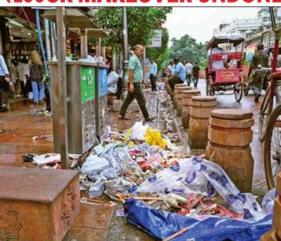
In Sept 2021, Chandni Chowk got a ₹100cr makeover, making it more visitor-friendly and clean. Three years later, there are overflowing litter bins, garbage outside shops, broken tiles, drain covers and bollards, cables hanging over the road and homeless people on the central verge. PWD and MCD are fighting over who's responsible for cleaning the area after the maintenance agency's contract expired on Sept 7 | P 4
