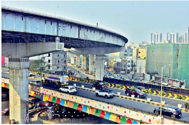
The six-lane flyover from ORR to Kondapur under construction. — R. PAVAN
