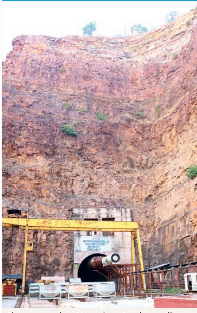
The entrance to the SLBC tunnel near Domalapenta village. — BY ARRANGEMENT
