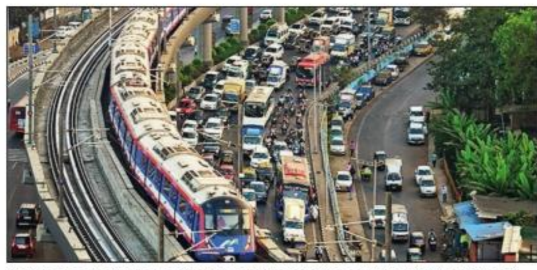
Systra has designed and overseen the Metro construction in Mumbai
