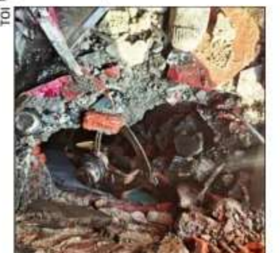
The third floor, where the blast occurred, was reduced to rubble
