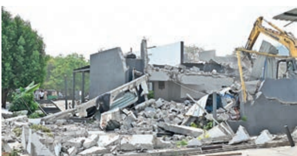
The unauthorised structures on government land at Hafeezpet that were razed by HYDRAA.
