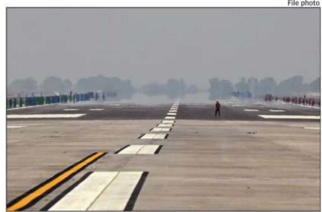
UP has imposed a fine of ₹10L per day on YIAPL from Jan 1 for the delay
