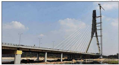
File photo Officials say assessment of the lift system is being undertaken alongside wider efforts to evaluate and restore various components of the bridge
