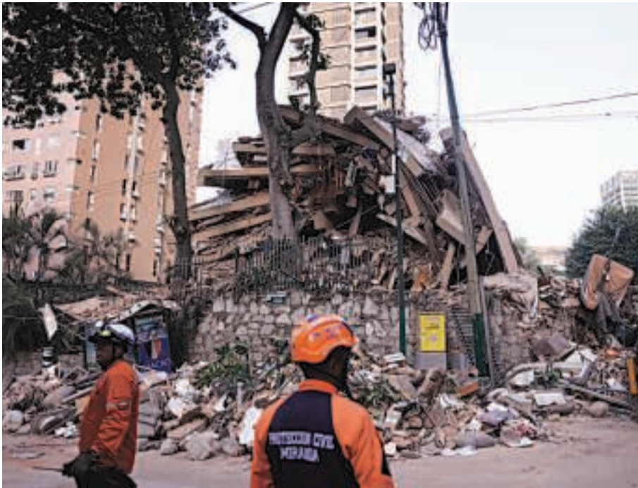
Emergency services work at the site of a collapsed building after earthquakes hit Venezuela on Thursday PHOTO: REUTERS
