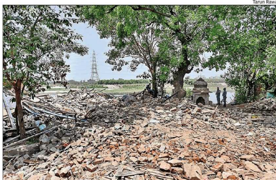
The demolition follows directions of Delhi High Court and National Green Tribunal mandating the removal of encroachments from the ecologically sensitive O-Zone floodplain
