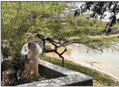
LG inspected ongoing work at the lake
